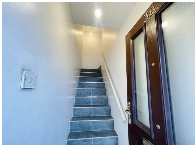
Composite front door. Steps to first floor.
