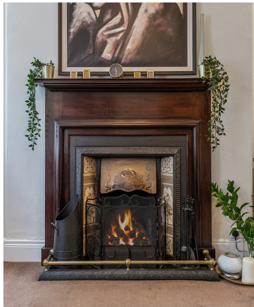
Period fireplace with cast iron and tiled inset
