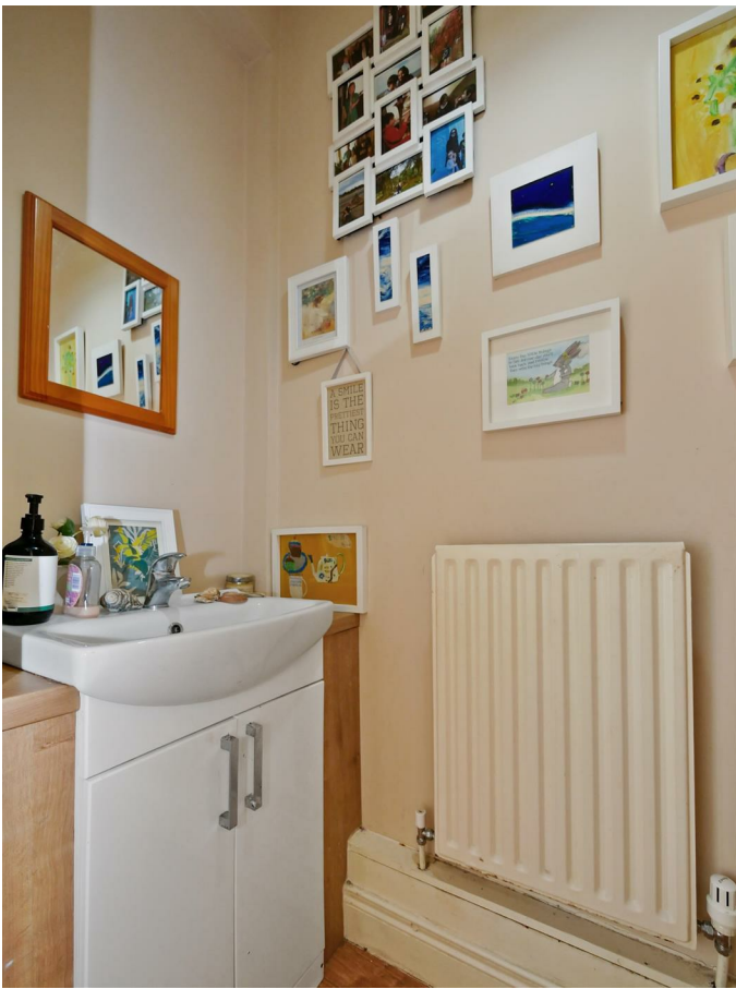
Sink unit & Low flush w.c
