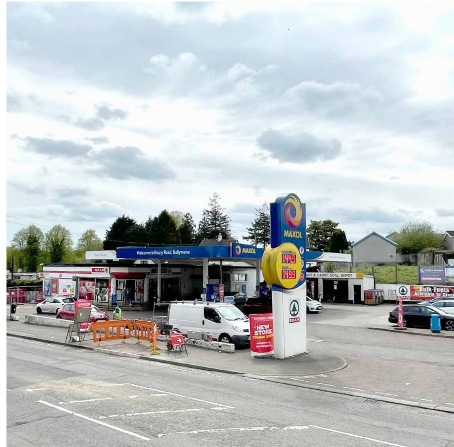
Construction works have commenced to the rear of the existing store.
