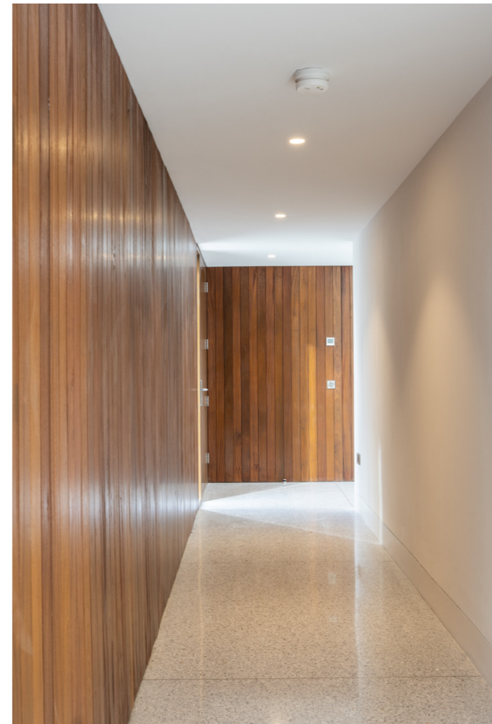
Iroko pannelled inner hallway
