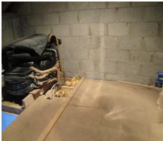
floor space of Attic.
