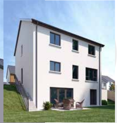
View of rear of site 10
