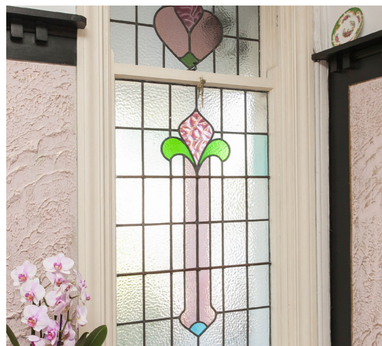
Stained leaded glass window details
