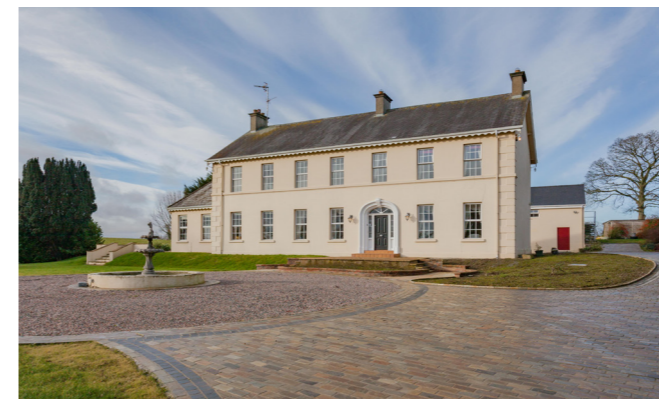
Front facade in style of traditional country house
