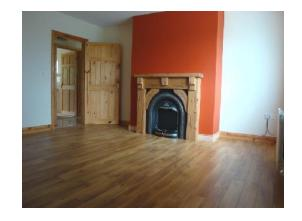
Timber finished fire surround and cast iron inset provided to open grate.
