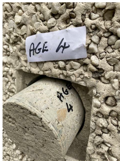
Photograph No 4 – View of northwest facing gable showing location of Core Ref AGE 4
