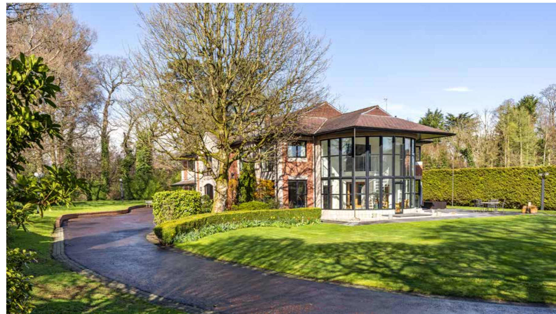
190 Upper Malone Road, Dunmurry
