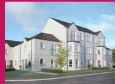
SHIMNA MILE Newcastle BT33 0TQ
