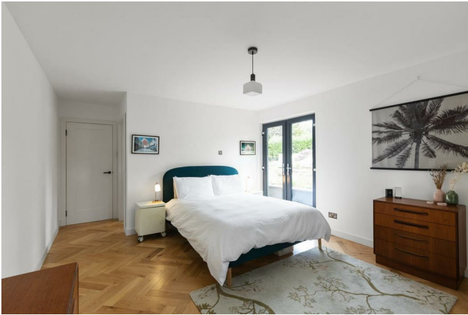
Oak flooring laid in herringbone style.
