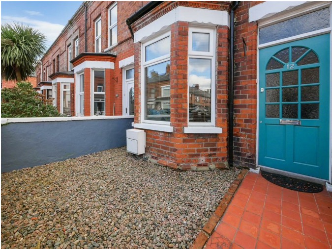
Loose stone area to the front.
