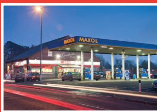
Spar Filling Station
